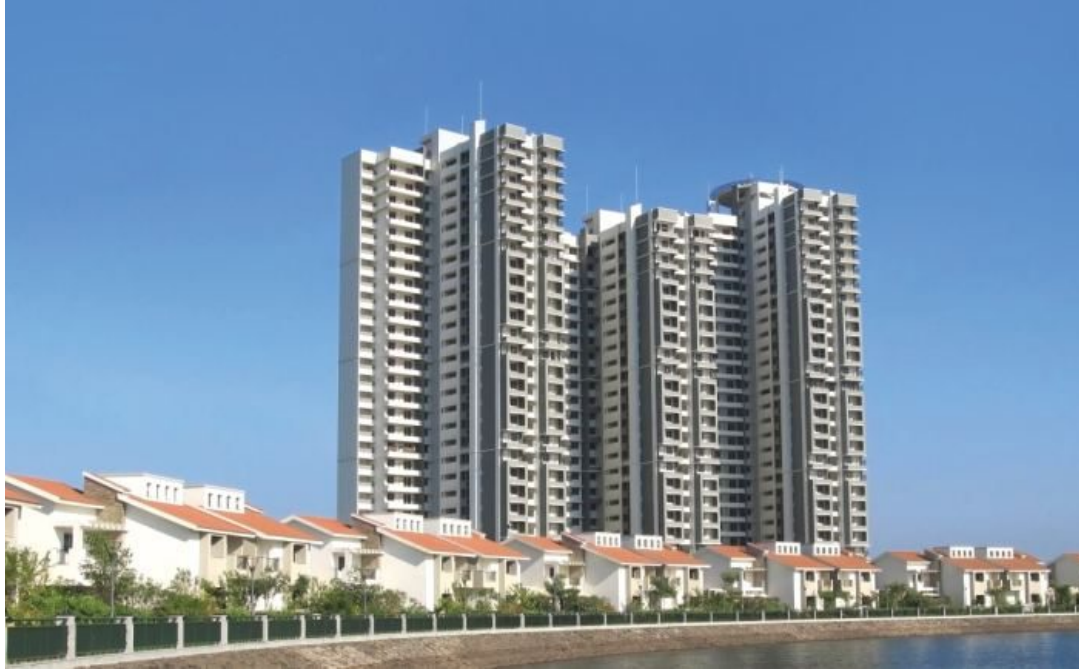
Sobha City, Thrissur: A 55 acre integrated township including a 6.5 acre lake - one of the biggest rainwater harvesting facilities in the country
